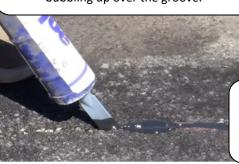
We modified the sealant tip for them so that the sealant would flow easier. Use a Sealant Tip and
