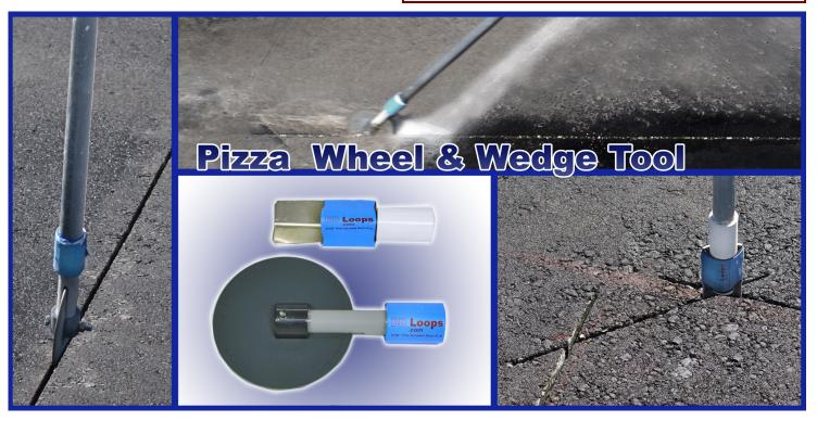
Easily roll Saw-Cut Loops to the bottom of the groove while standing by using the BD Loops Pizza Wheel & Wedge Tool. Many loop installers use screwdrivers, paint mixers, sticks, or other tools to stuff saw-cut loops into saw-cut grooves. Those tools are not only inefficient, but some can knick the loop wire and cause the loop to short to ground.
