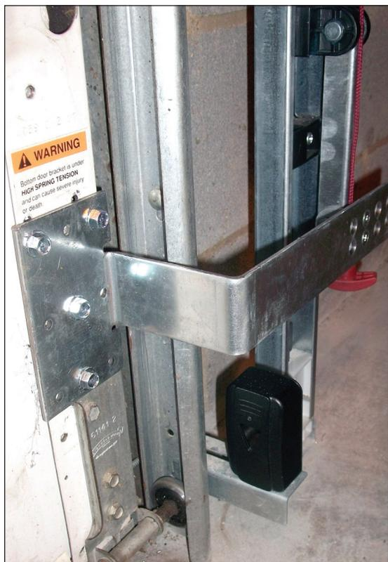
2. Install the vertical mount bracket to the lower inside edge of the bottom section.
