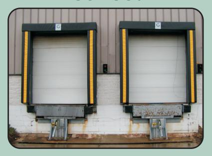
Standard Dock Seal compresses and form a positive seal between building and vehicle. Provides an energy-efficient, weather tight seal designed to withstand constant abuse of trucks, extreme temperature and weather. In addition, regulating theft and security.
