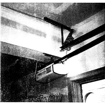
SIDE MOUNT ARMS are available in right hand and left hand assemblies and can be used on most any torsion spring doors.
