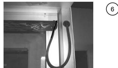
4. Hold the SuperScan extrusion up to the top of the door. Insure that the extrusion is oriented correctly as shown below.
